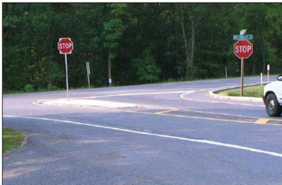
Figure 15 Example of Median on Minor Street Approach (Source: https://www.columbus.gov/uploadedfiles%5CPublic_Service%5CTransportation%5CMobility%5CEstimated%20Costs%20FINAL.pdf )
