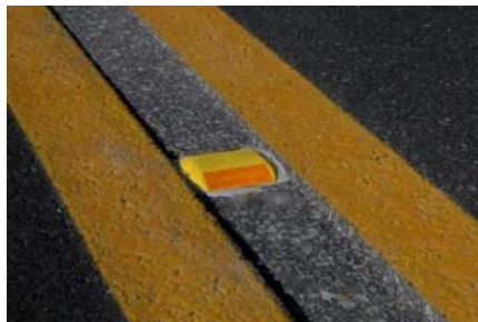
Figure 14 Example of Inlaid (Recessed) Raised Pavement Markers (Source: http://safety.fhwa.dot.gov/roadwaysafetyawards/2013/ )
